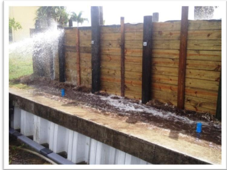
Photo of inclinometers in place (blue)
